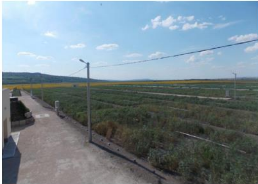
Figure 9-6 – Pictures from the Orhei WWTP
