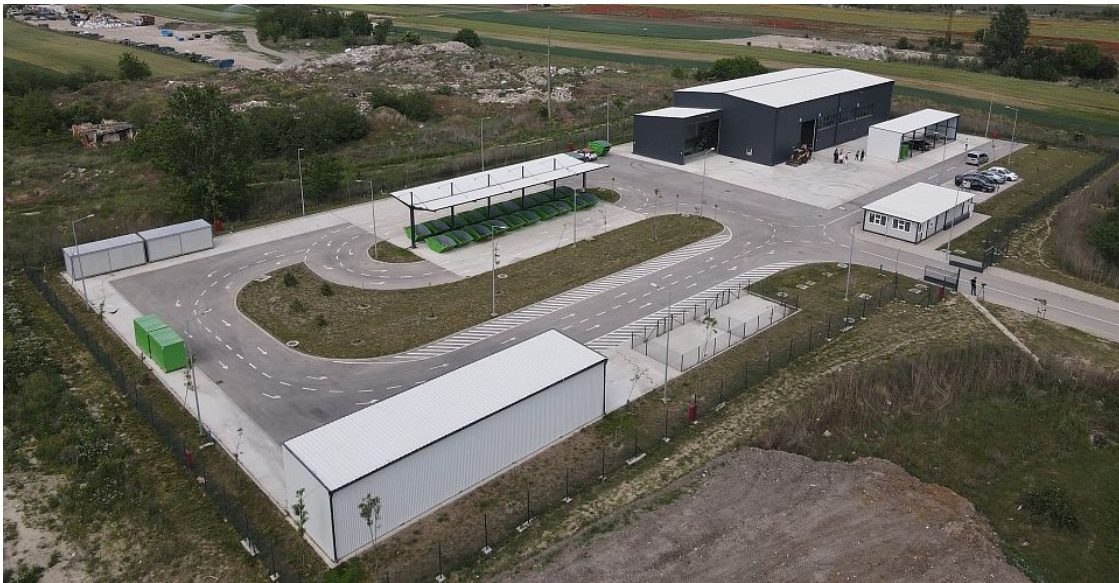
Figure 24 Recently opened recycling yard in Novi Sad 14
