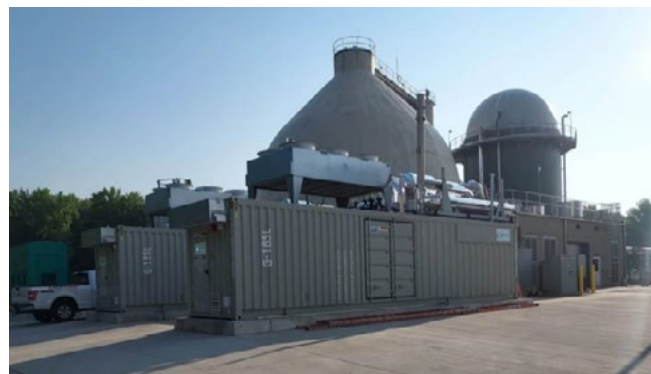
Photo 4.6 Example of the CHP unit within the WWTP
