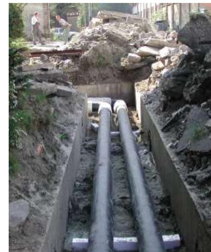
*Photo 8. Installing new district heating pipes*
